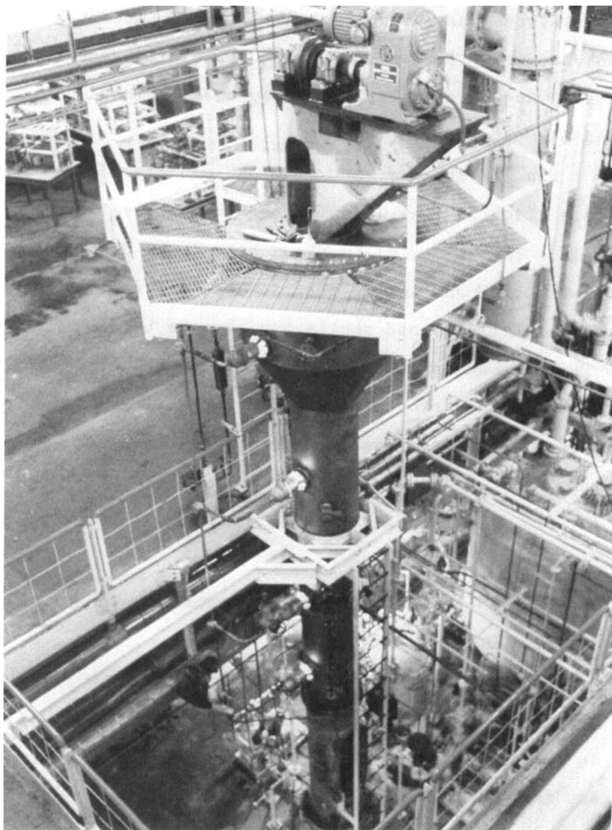
FIGURE 11. 24-inch diameter column for high interfacial tension system.
