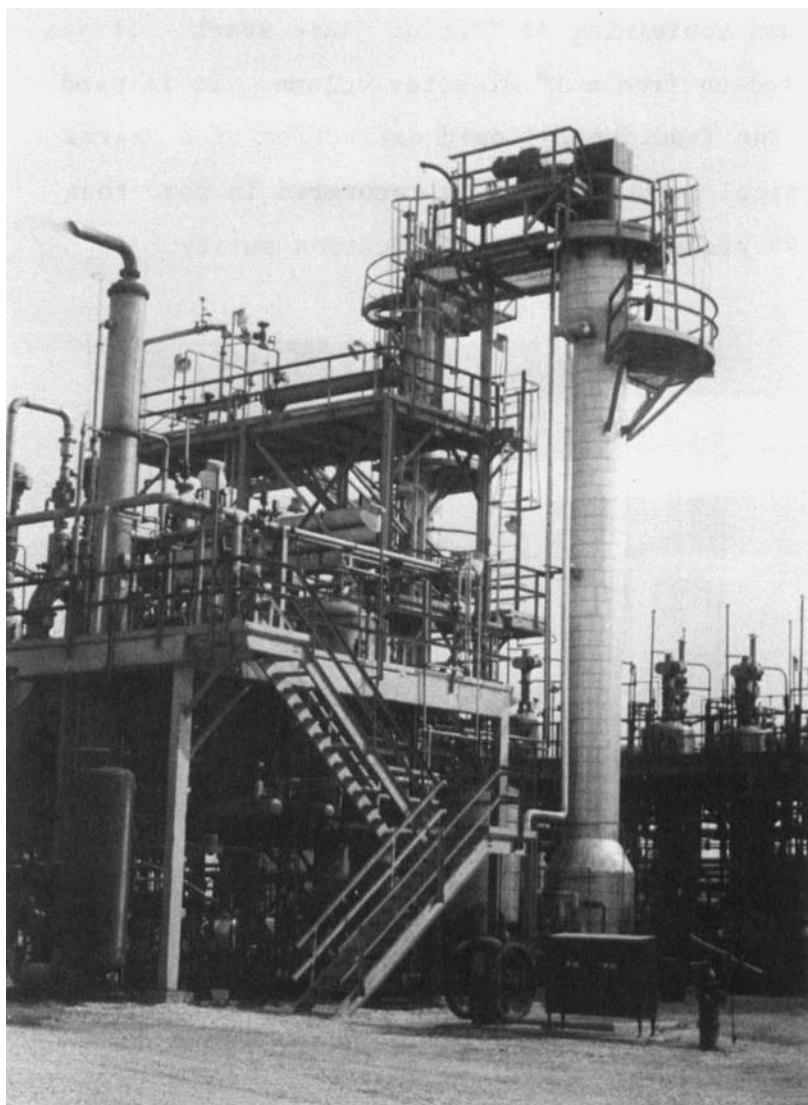
FIGURE 8. 40-inch diameter column containing 32 feet of plate stack.
